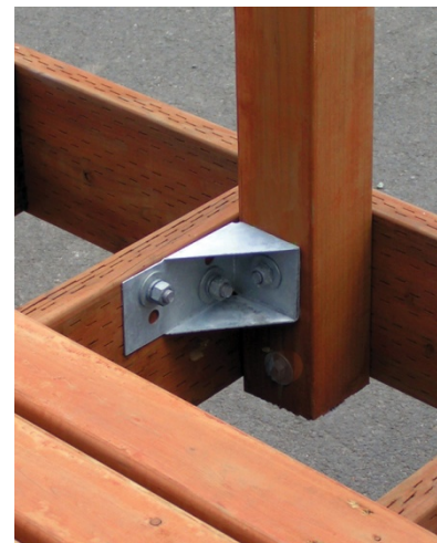
FIGURE 2—TYPICAL BRACKET INSTALLATION
